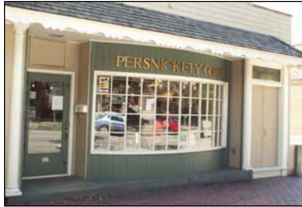
Figure 4 - Wall sign showing proper location above storefront
