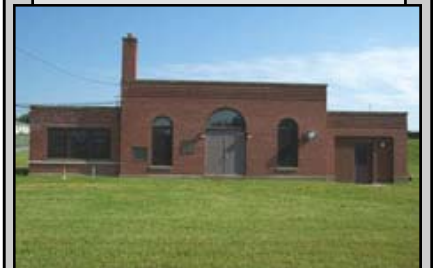
Facility #3 (Ground Water) .864 MGD by Permit
