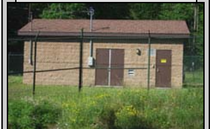
Facility #2 (Ground Water) 1.152 MGD by Permit
