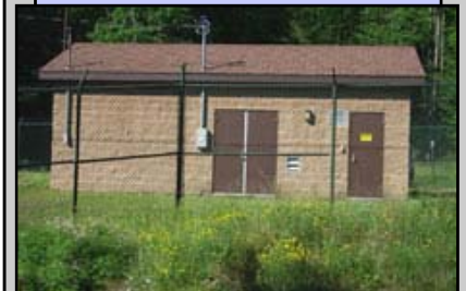
Facility #2 (Ground Water) 1.152 MGD by Permit
