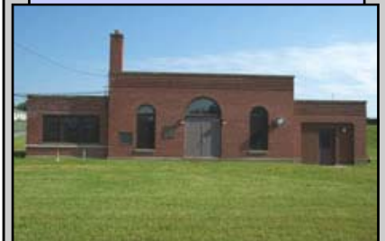
Facility #3 (Ground Water) .864 MGD by Permit
